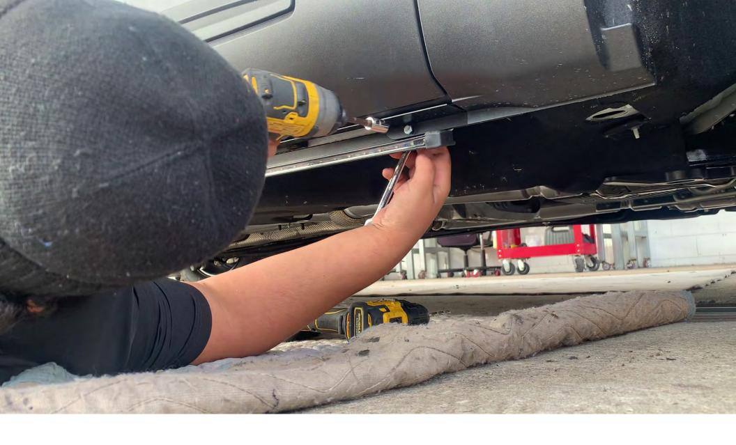
7. Place the HG2 Siderunner in between the plastic and metal tabs and bolt it in with a nut on the other end (repeat on other two tabs)
