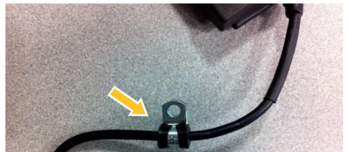
Fasten wire stress-relief clamp to underside of vehicle in a suitable location using self-tapping sheet metal screw.
